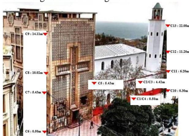
Figure 1 - Location of the sensors on the structures.
