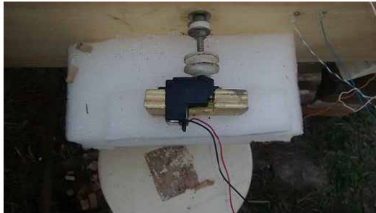
Figure 4. Servo motor used to open /close the air admittance valve.
