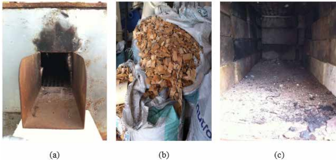
Figure 2. (a) Combustion chamber and furnace grate; (b) Chip; (c) Ash warehouse.
